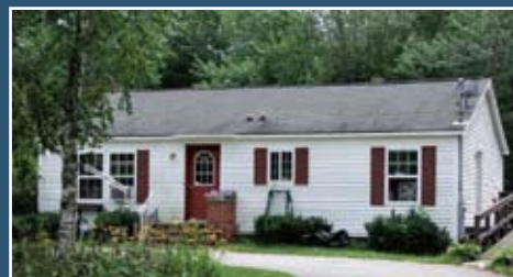
542 Maine Street, Stoneham
